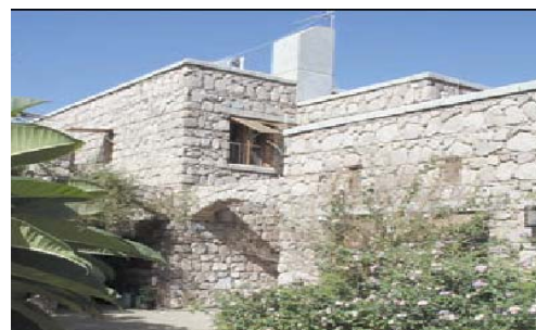
Figure 5-13 Local granite used in Aqaba. Source: (CSBE, 2001)
