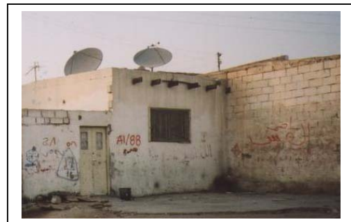
Figure 5-9 One of the most basic construction styles in Aqaba
