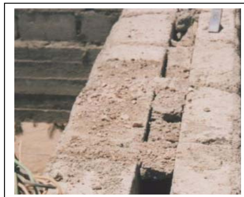
Figure 5-12 Rubble filled cavity walls, planned KFC restaurant, Aqaba
