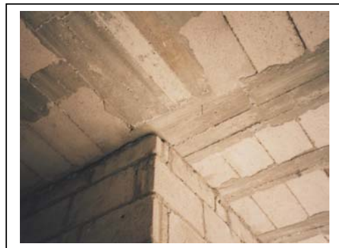
Figure 5-11 The only residential roofing construction style used in Aqaba today
