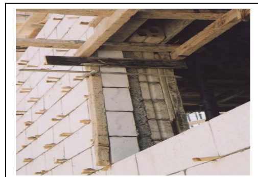
Figure 5-10 The standard high-end construction style using Ma'an limestone
