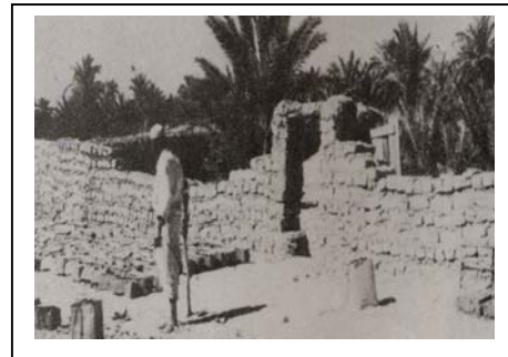
Figure 5-1 Aqaba mud bricks in construction [Image courtesy of Khammash]
