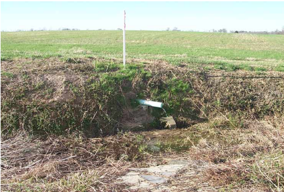
Figure 18: Tile drainage (source: www.cyber-diver.com/egypt_map.htm . last accessed on November 15 th , 2006).
