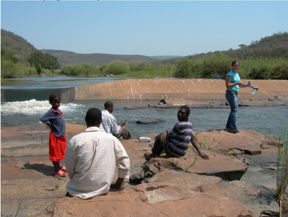
Site 5 – Sampling was made just downstream the centre of the weir.
