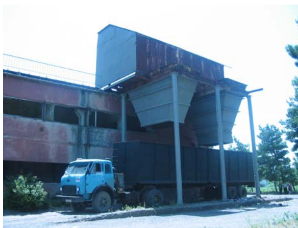
Figure 8-2. Loading station at Ponichala, Tbilisi
