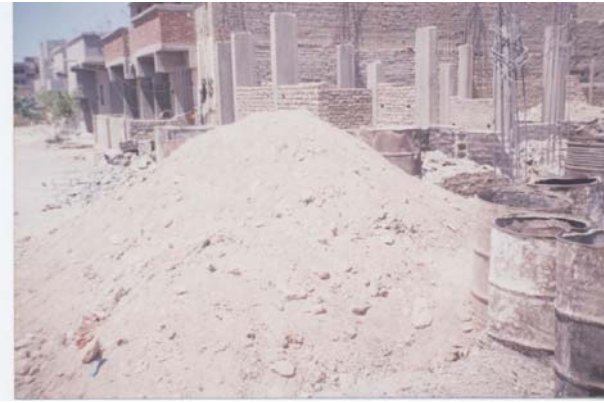
Figure 13 C&D waste accumulations inside Quseir City
