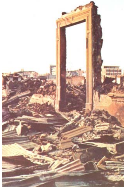
Figure 7.1 Gate standing tall in the 1972 earthquake.
