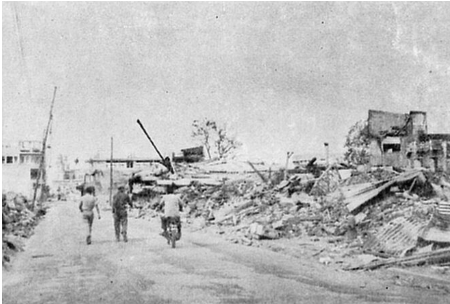
Figure 1.1 A collapsed five-story building in the 1972 earthquake.
