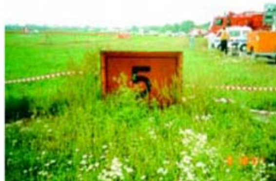
Photograph 12 - Location sign at TWY R5 entrance (exiting North apron).
