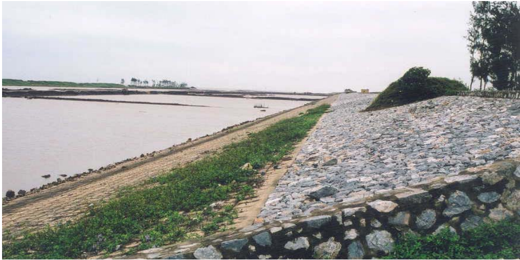
Figure 3.6 The second line of rock-reinforced dikes at Hai Hau Beach.
