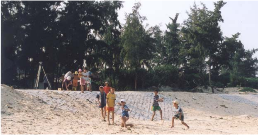
Figure 3.12 Recently constructed revetment at Ly Hoa Beach.
