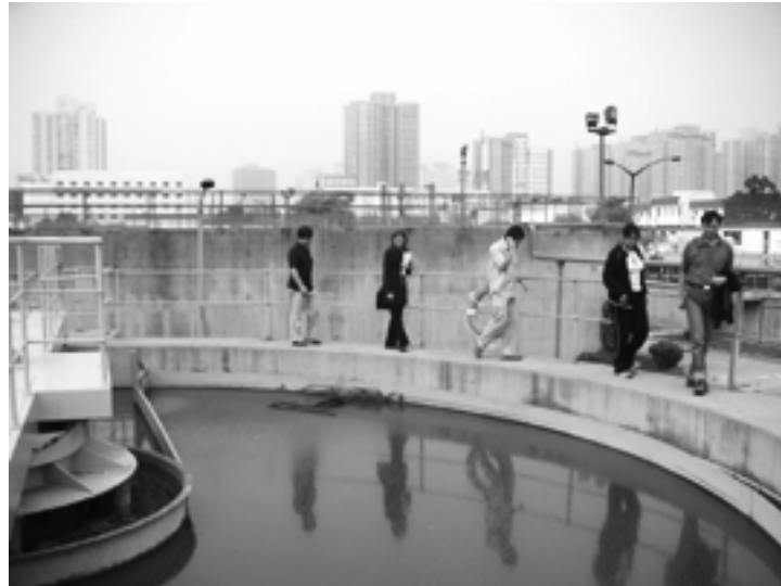
Figure 6 Thickening tank at Fangzhuang Sewage Treatment Plant with the surrounding housing area.
