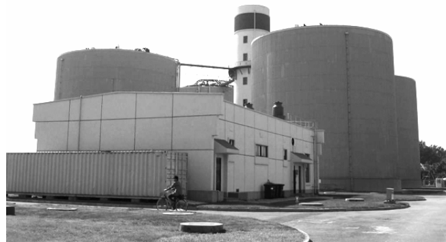
Figure 8 Digestion chambers at Gaobeidian Sewage Treatment Plant.
