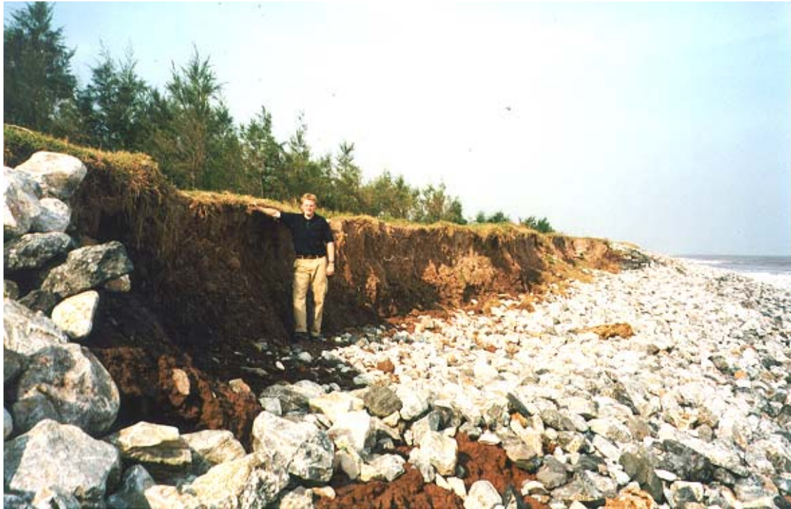
Figure 3.8 Severely eroded dike with planted Casuarina trees at Hai Hau beach.
