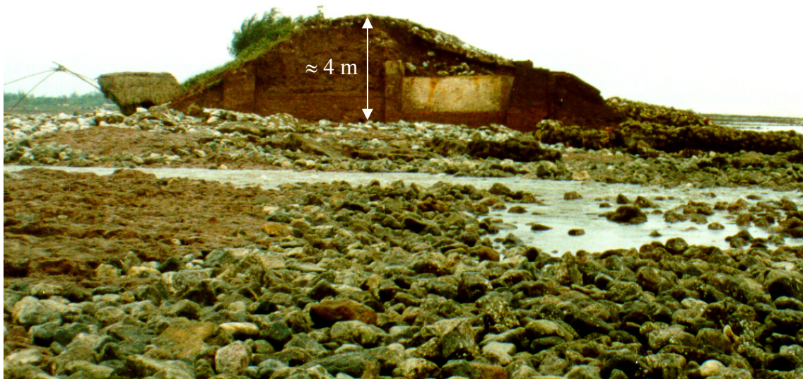
Figure 3.9 Characteristic cross-section of an eroded dike near Van Ly village, (former shrimp farm to the left; open sea to the right).
