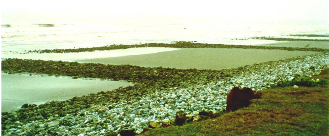
Figure 4.3 Groins with insignificant impact on the longshore sediment transport at Van Ly beach (photos taken at low water).
