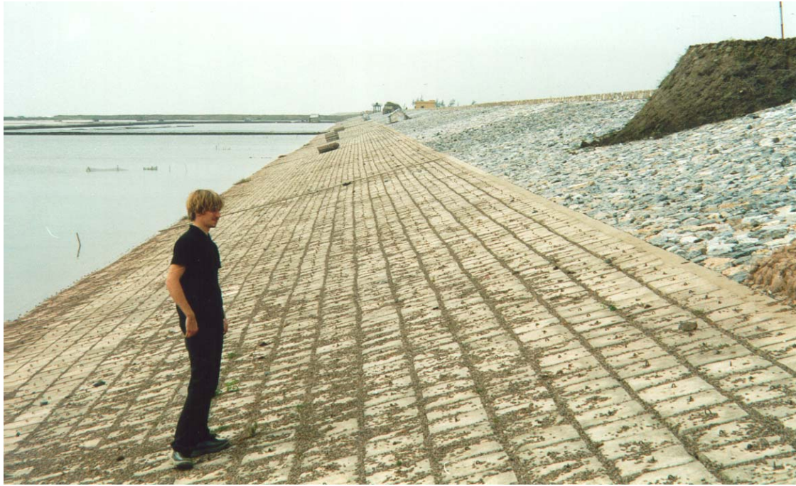
Figure 4.2 Concrete revetments on a second sea dike in Van Ly.
