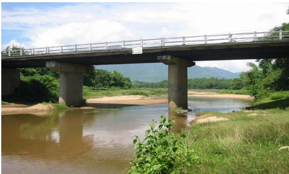
Figure 2.1.1: The bridge at Hoa Phu.
