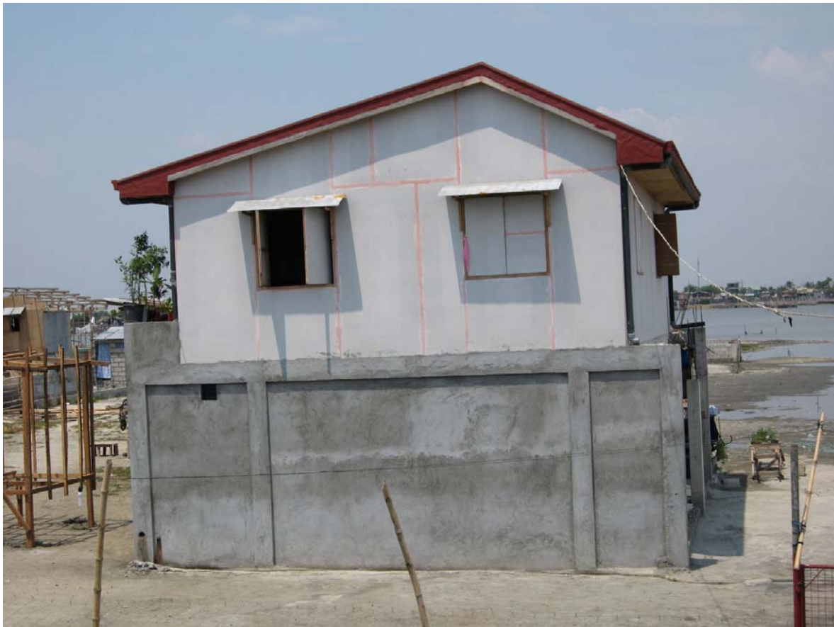
Fig. 23 Solid foundation, Sanagmana, 2007-04-14
