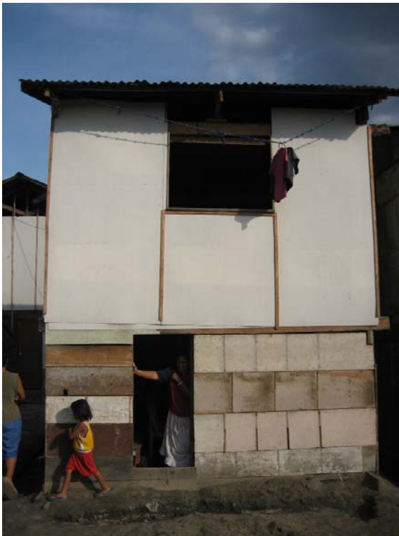
Fig. 47 Family K's house, Sanagmana, 2007-04-28
