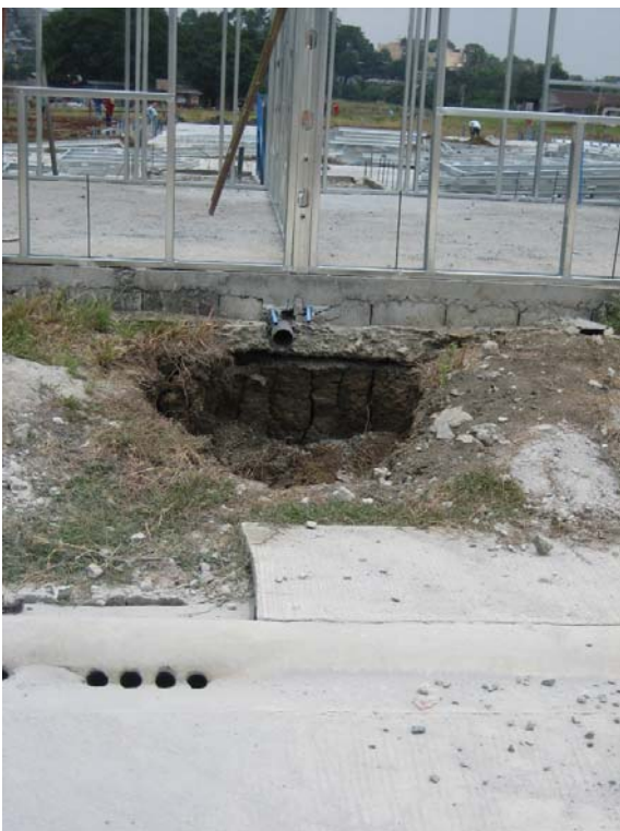
Fig. 7 Preparation for the septic tank, Baguio, 2007-05-02
