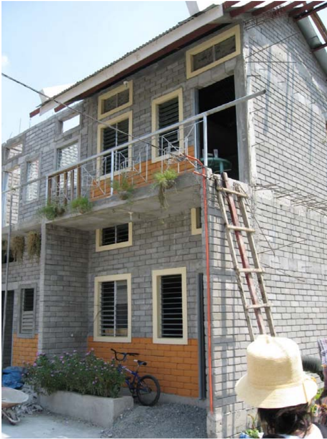
Fig. 15 Ready construction, Pasay, 2007-04-17
