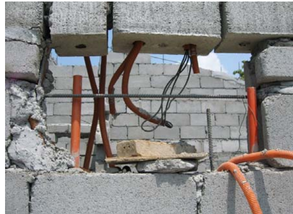
Fig. 36 Reinforcement and installation, Pasay, 2007-04-18
