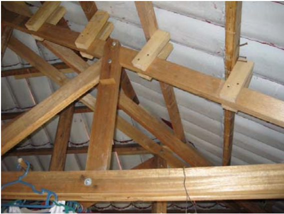
Fig. 29 Roof construction, Sanagmana, 2007-04-14
