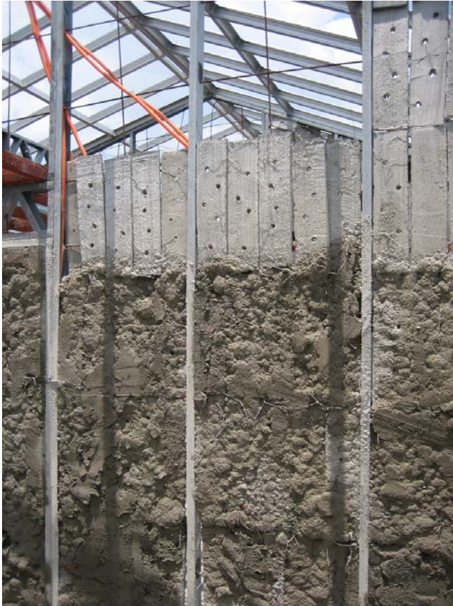
Fig. 4 The construction, Baguio, 2007-05-02
