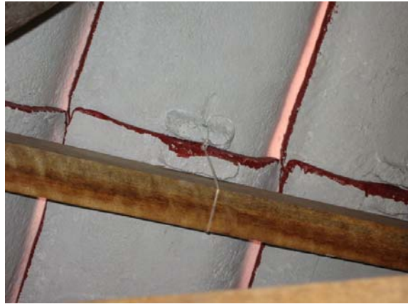
Fig. 30 Tile anchored with nylon, Sanagmana, 2007-04-14
