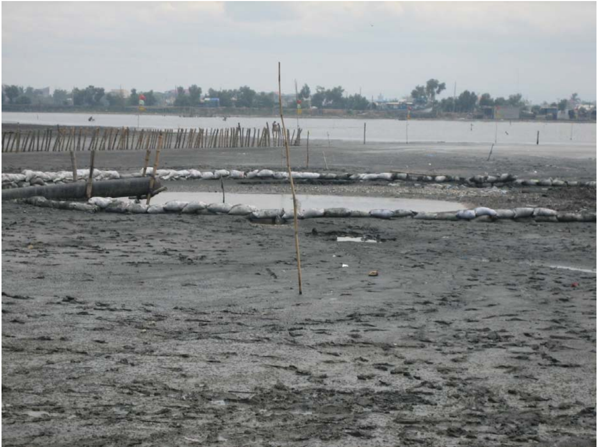
Fig. 24 Filling up the land with silt, Sanagmana, 2007-04-28
