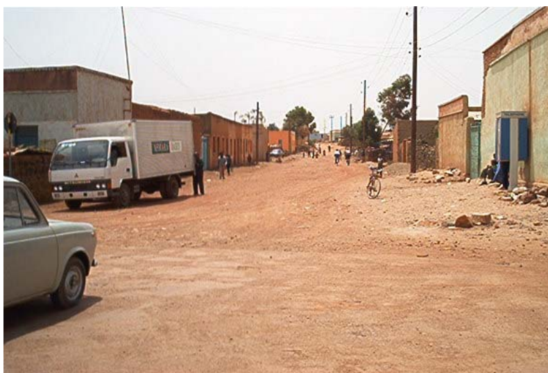
Figure 3.9 Typically unpaved road in Asmara
