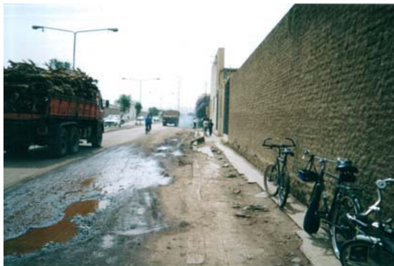
Figure 3.7 Road in poor condition
