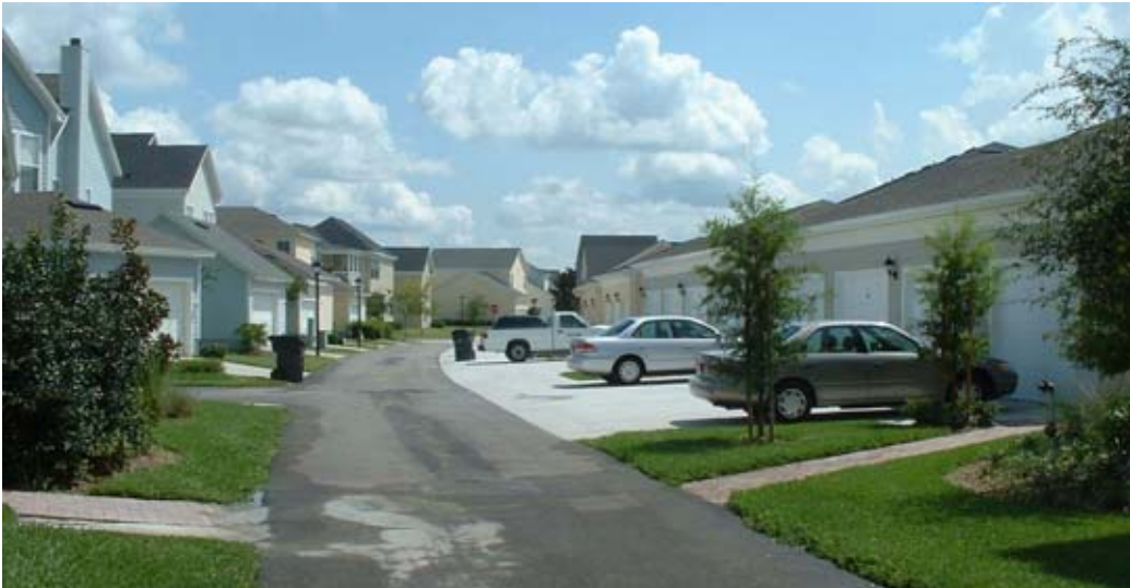
Illustration 4.3 Typical backyard alley with garages
