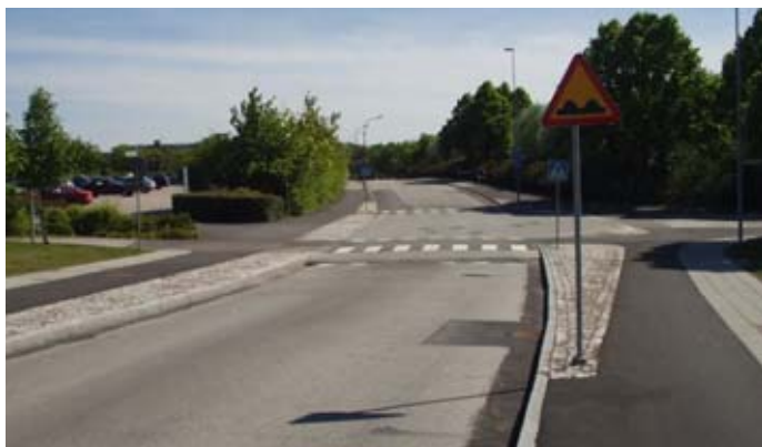
Figure 12 Flat top hump at Ole Römers väg, looking south
