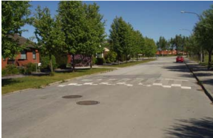
Figure 6 Hump at Kulgränden, looking north
