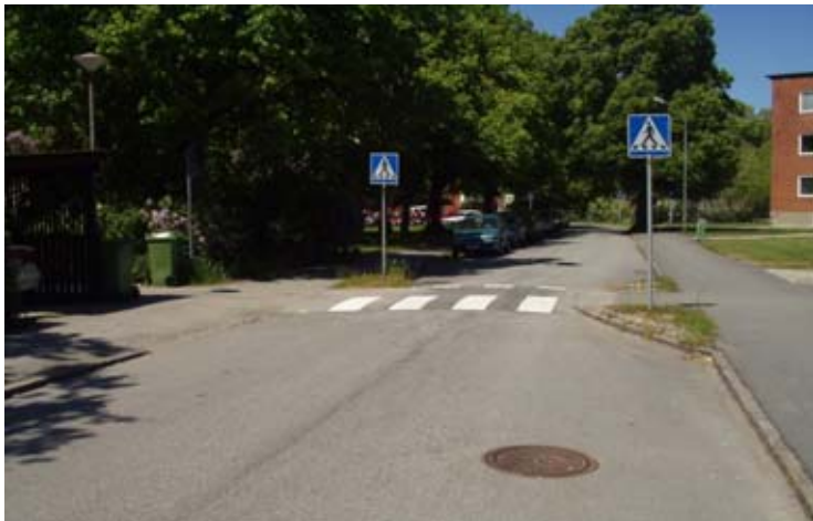
Figure 5 Road hump nr. 3 at Kakelvägen, looking north-west
