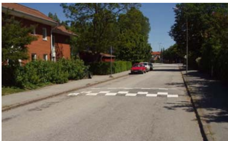
Figure 10 Hump nr. 1 at Måsvägen, looking south-west
