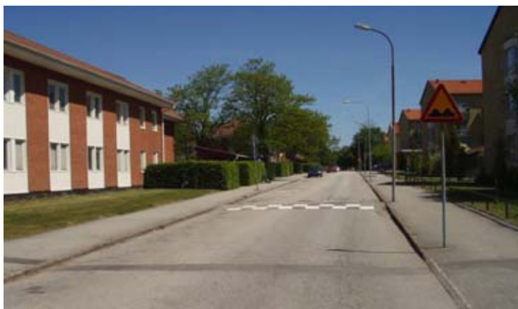
Figure 11 Hump nr. 2 at Måsvägen, looking north-east
