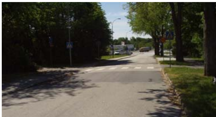
Figure 1 Flat top hump at Bondevägen, looking south
