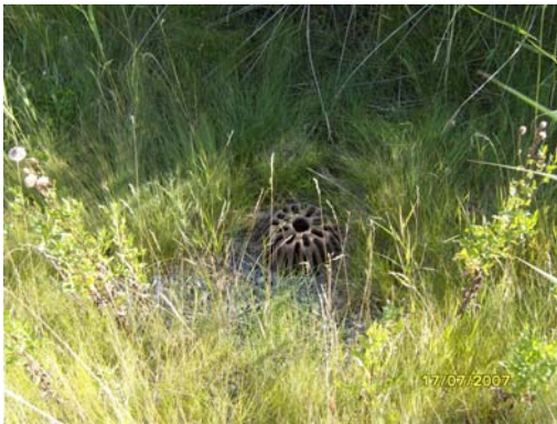
Figur 4.25 Infiltrationsbrunnar placerades i diket (Foto: Zainab Mousa)
