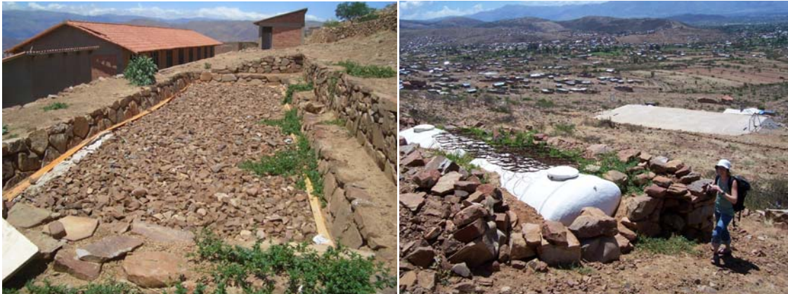
Figure 22. The wetland (left) and potable water tanks (right) at San Nicholas in Pukara.
