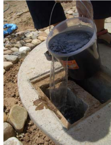
Figure 26. Adding the salt solution to the septic tank.
