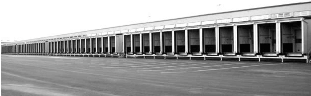
Figure 29 One of the largest logistic centers in Sweden, all docking equipment delivered by Crawford. (Internal documentation 2009)
