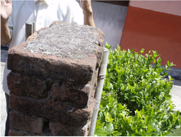
Fig. 2.1 Bamboo attached to a soil brick wall to make it earthquake resistant.
