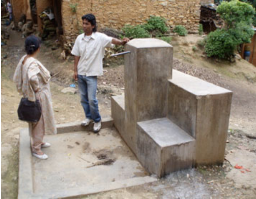
Fig. 6.6 Showing one of the three water taps in the village.
