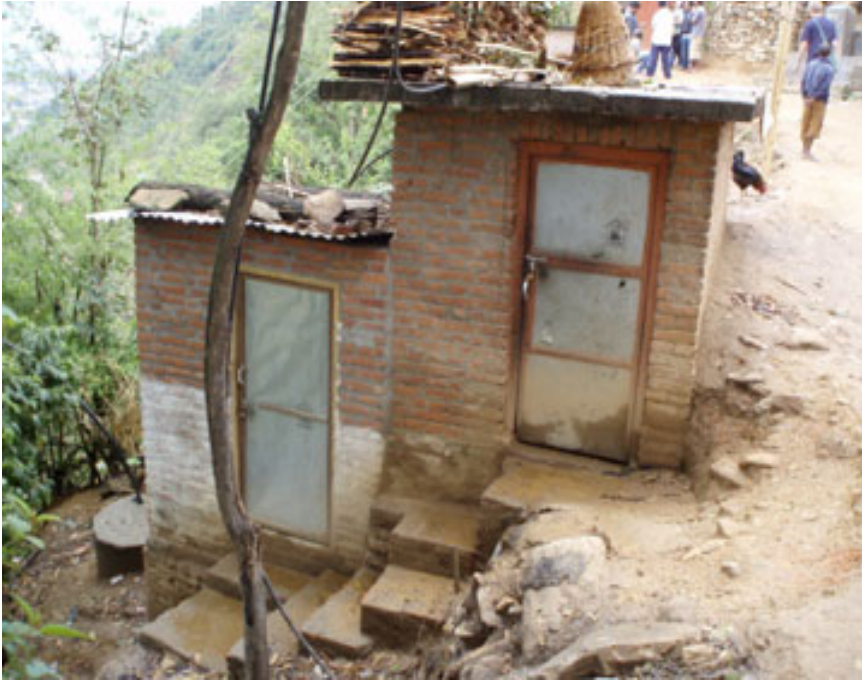
Fig. 6.7 One of the toilets from an aid organisation in the village.
