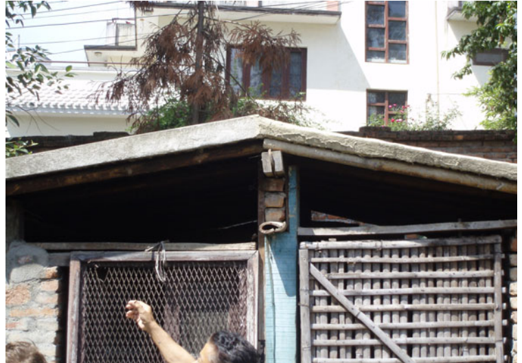
Fig. 2.2 A soil roof.
