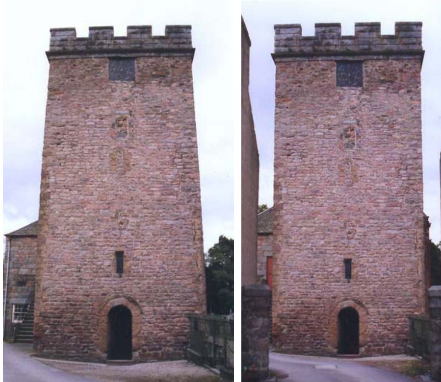
Figure 4: The west elevation of the tower. The left photograph is taken from about 6 metres while the right is taken from 24 metres. It has been taken with a straight on view, without obliqueness. Photograph by Gertie Ericsson 1997.
