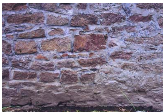
Figure 16: Different types of stones, limemortar and repointed cement. Photograph by Gertie Ericsson 1997.
