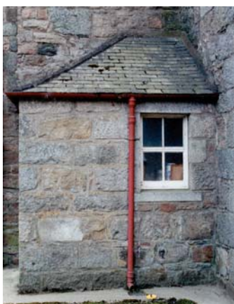
Figure 31: The toilet on the north side of the complex. Photograph by Gertie Ericsson 1997.
