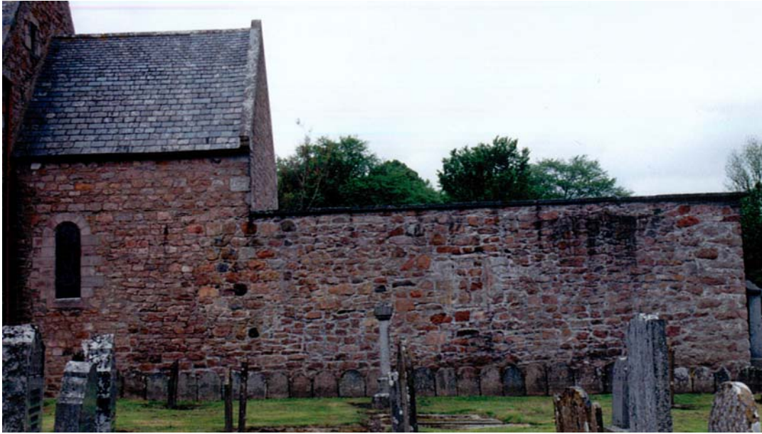
Figure 26: The extended south elevation of the chancel. Photograph by Gertie Ericsson 1997.
