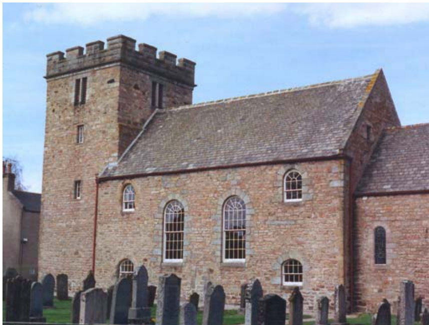
Figure 24: South elevation of tower and nave. Photograph by Gertie Ericsson 1997.
