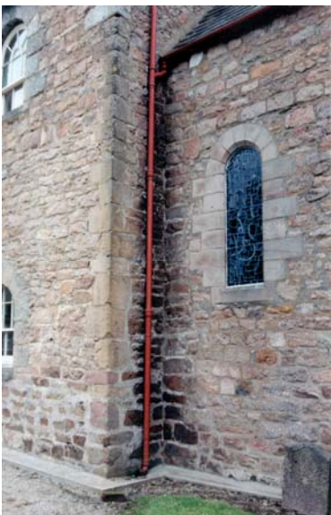
Figure 28: Masonry of phase one, southwest extent of chancel. Photograph by Gertie Ericsson 1997.
