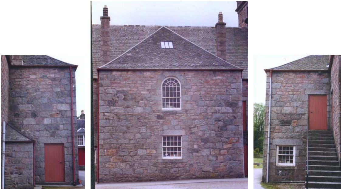
Figure 30: The modern north aisle. The east, north and east elevations. Photograph by Gertie Ericsson 1997.
