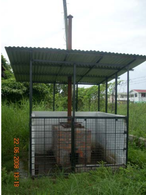
Newly constructed De Montfort incinerator used for incineration of sharp waste at the West Demerara Regional Hospital
