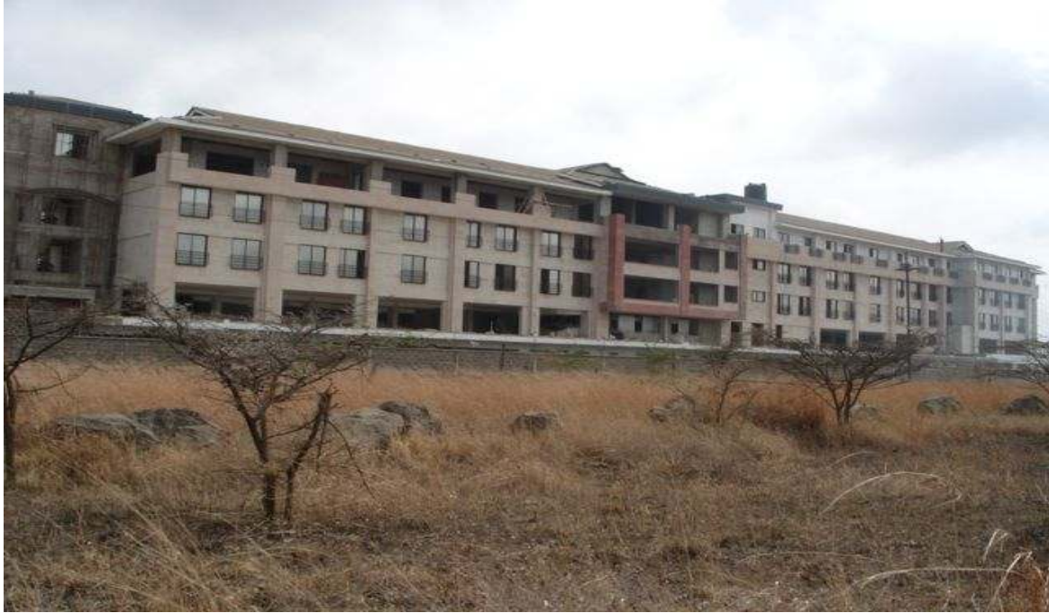
A hotel construction
