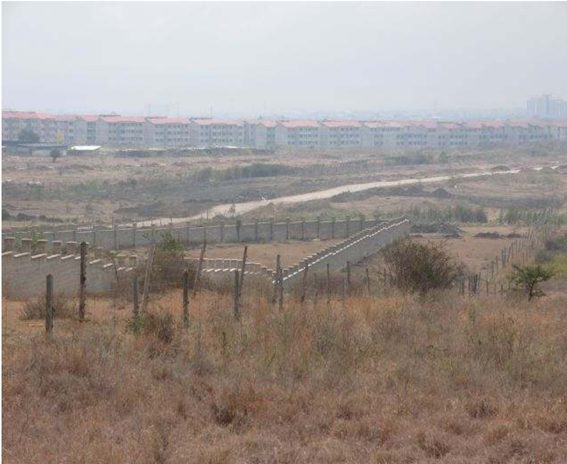
Houses being constructed
