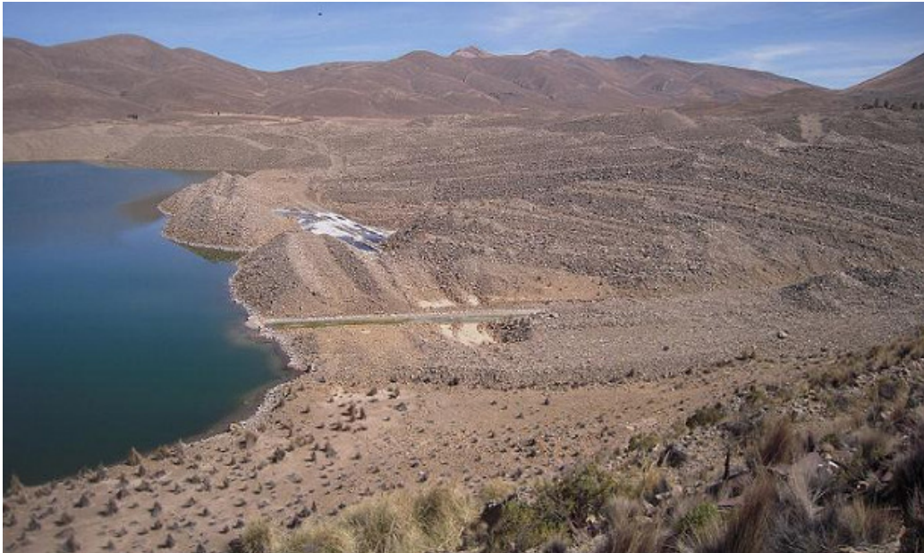
Figure 5-2. Photograph showing the massive tailings including its dam in the Antequera sub basin. The dam is holding a pH of 3.07 (Ekdahl, 2007).
