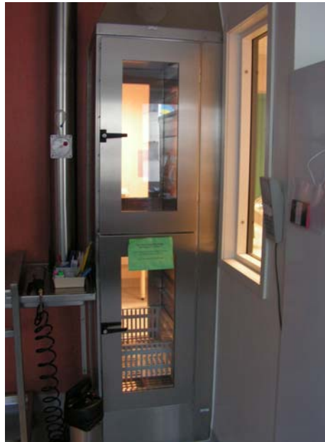
Figure 2: The sterile cupboard between the drugs room and the preparation room
