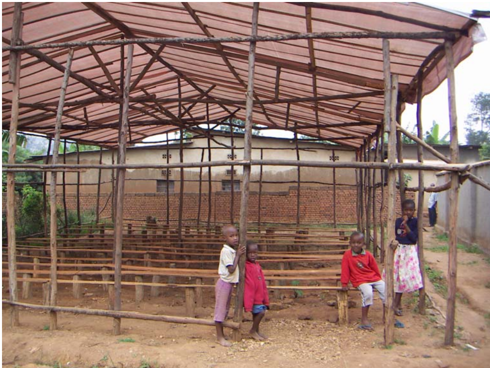
Gacaca courthouse in the outskirts of Kigali.
