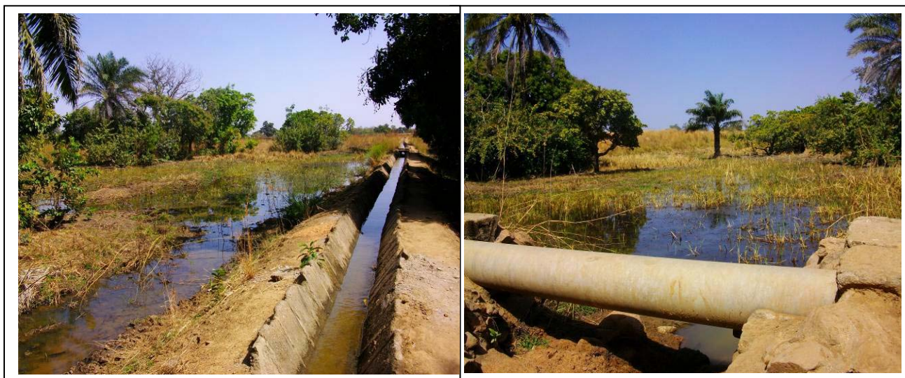
Plate 2 Pictures showing water wastage due to lack of water conservation at Kajelo Dam
