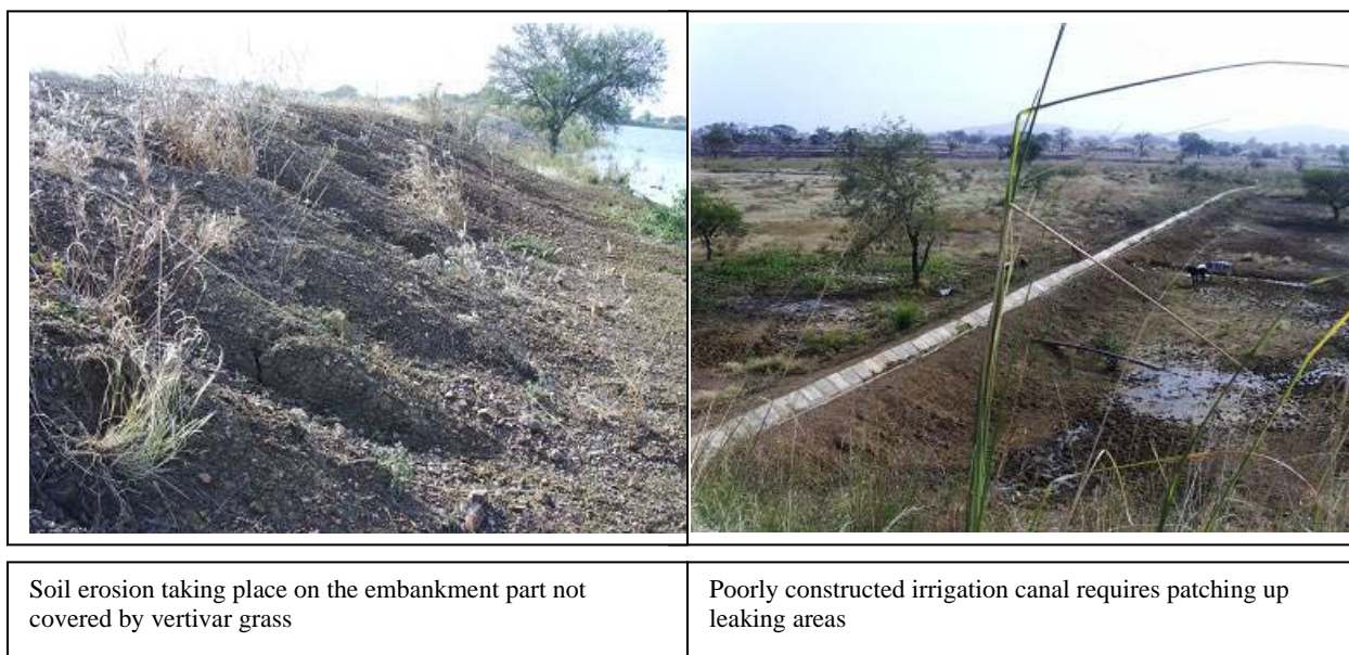
Plate 1 Pictures showing signs of soil erosion and a poorly constructed irrigation canal in Baare
