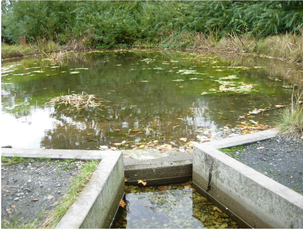
Picture (3). Pond 2 – the end of the Augustenborgs open storm water system (sampling point 4)
