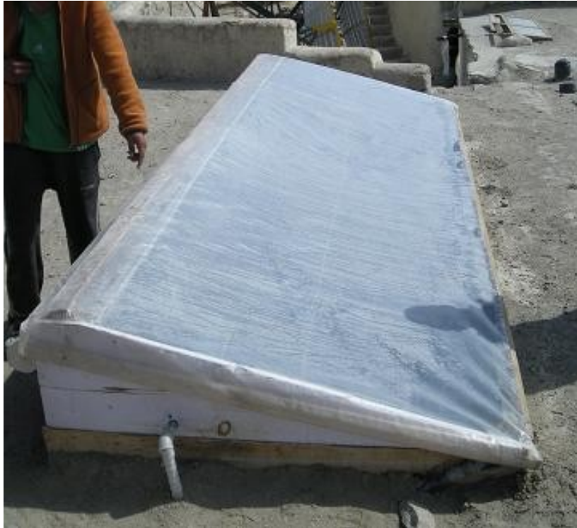
Fig. 7: Water heater at SECMOL Campus (photo by Sebastian Andersson).
