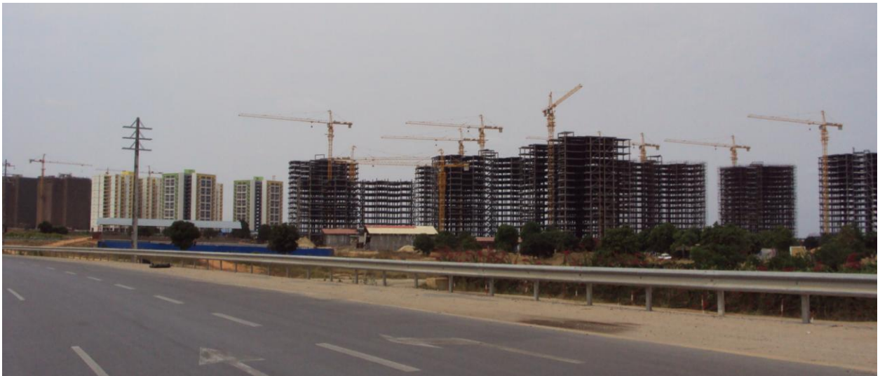
Apartment buildings and houses under construction in Luanda and Benguela
