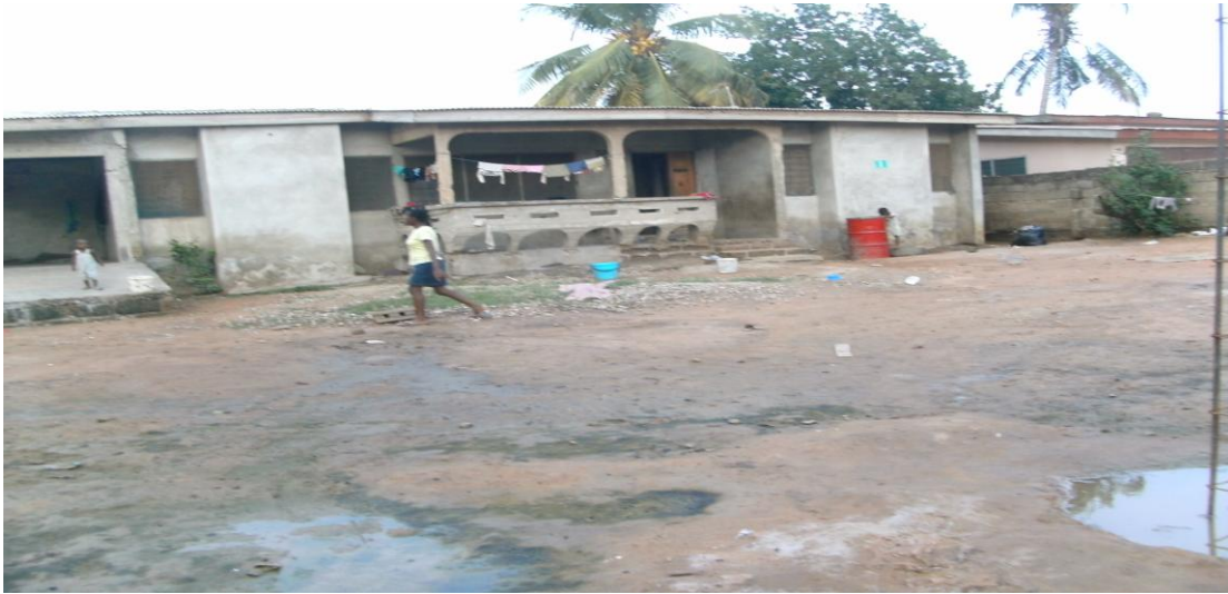
Figure 4.8: An uncompleted building been occupied by tenants at Awoshie
