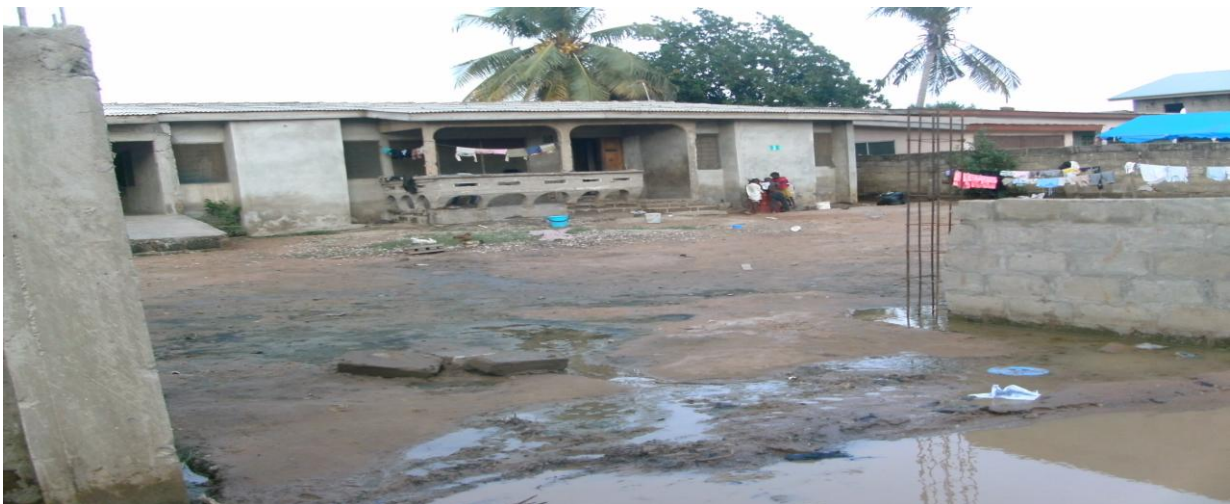
Figure 4.9A: An uncompleted building been occupied by tenants at Dome
