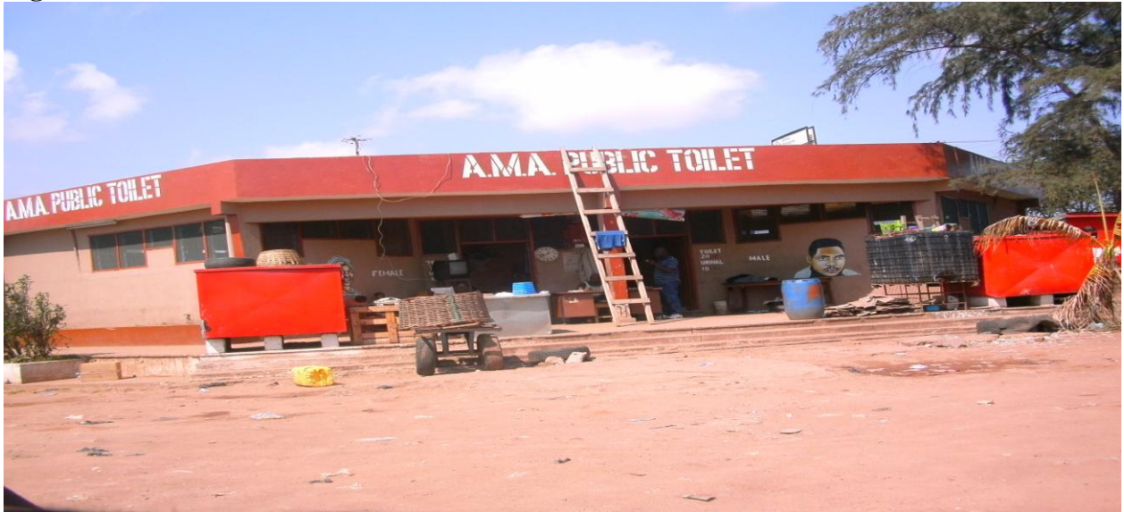
Figure 4.6A: Public Toilet at Abeka
