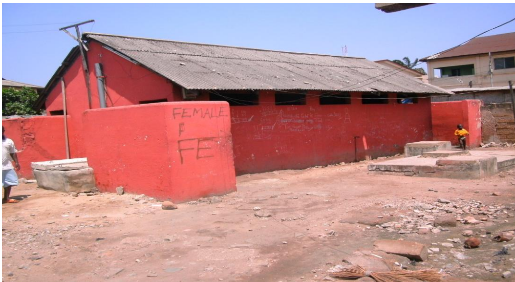
Figure 4.6B Public Toilet at Sukura
