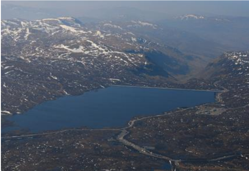
Figure 13. Glendoe Hydro electric scheme, Scotland. (Source: Scottish and Southern Energy, 2010).
