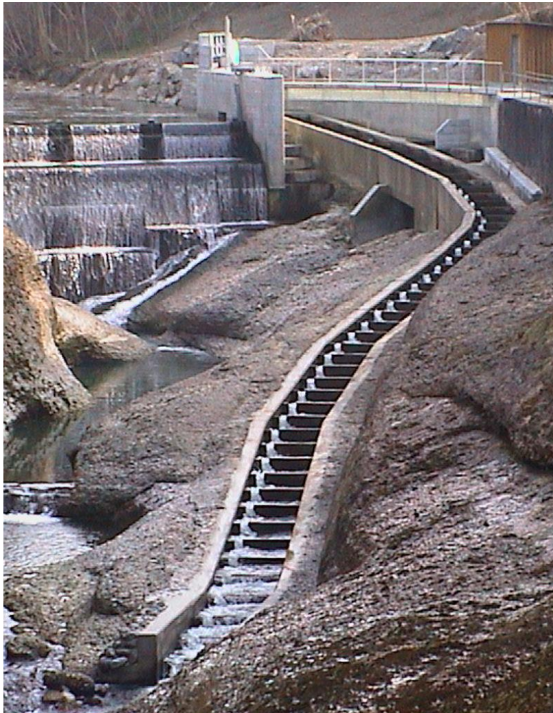
Figure 5. Fish ladder at Toggenburg, Switzerland. (Source: Hydroelectra AG, 2010)
