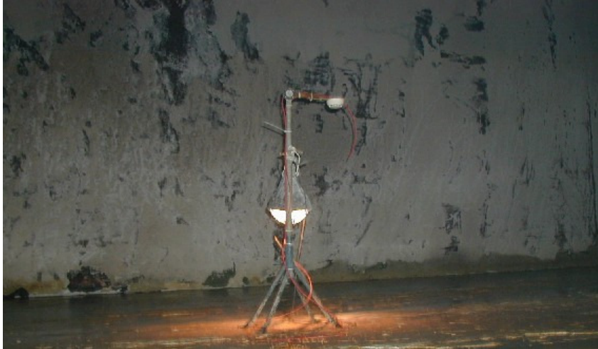
Figure 15 A stand with a smoke detector at approximately one meter above the ground inside the absorber.
