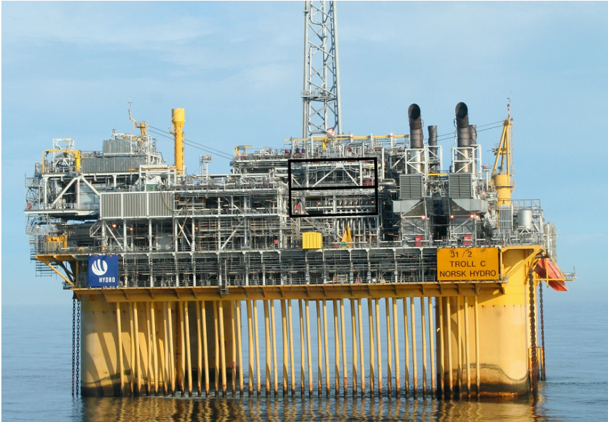
Figure 2.2 Troll C platform, square marks location for the new module (Aker Kværner AS, 2007a)
