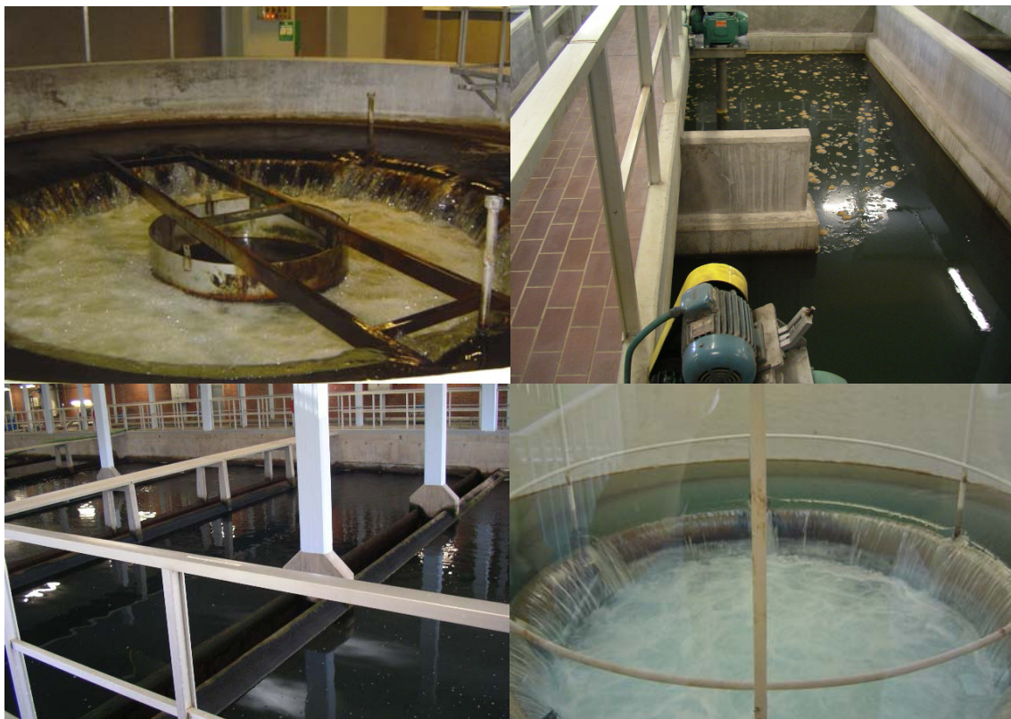
Figure 7. Upper left: raw water weir*. Upper right: flocculation mixing chamber. Lower left: GAC filters. Lower right: drinking water weir.
