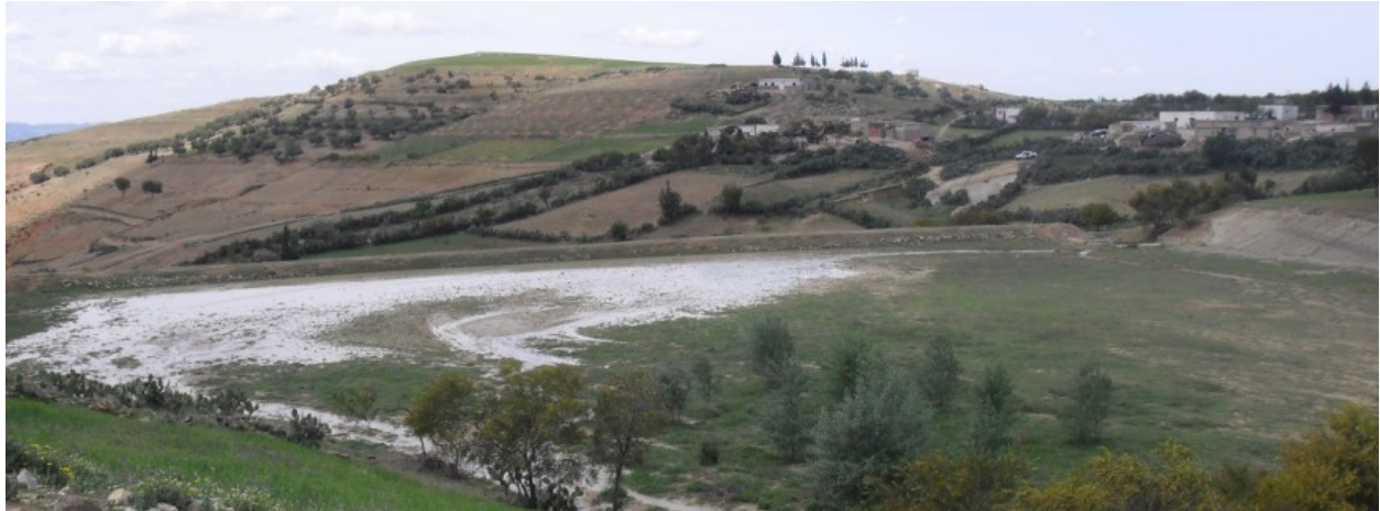
Figure 3; Silted reservoir in 'Sadine2' catchment in the Tunisian Dorsal. The reservoir has a capacity of 108 800 m 3 and was almost completely silted in approximately 10 years.
