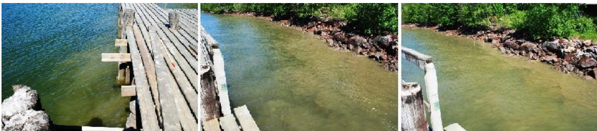
Figure 20 – Observed increase in SPM at Garn station. Pictures are taken after the wave systems of the ship Patria, passing in the downstream direction, had dissipated. The intake of water to Garn station is located at the beam in the left photo, some 10-11 metres off the bank, and is clearly affected by the increased load of TSS. Note the apparent decrease in SPM mass per unit volume of water with distance from the river bank (© Althage 2010).
