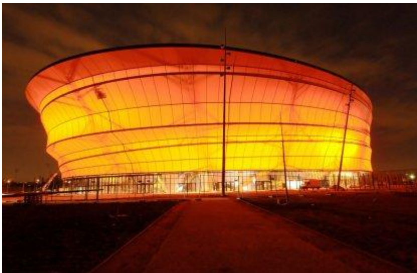
Figure 3. Zenith, a music palace able to contain 10 000 people, Strasbourg, France, silicone coated fibreglass, surface area: 12 000 m 2 , constructed in 2007. (4)
