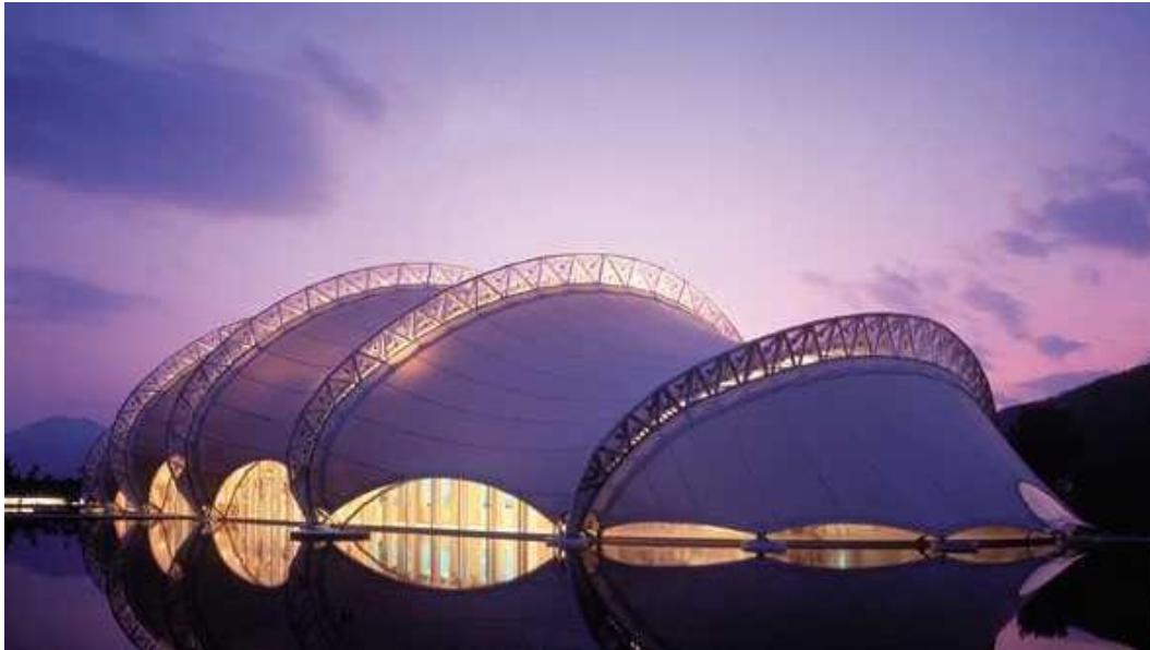
Figure 2. Centro M & G Ricerche, Venafro, Italia, PVC coated polyester, covered area 2 900 m 2 , constructed in 1991. (3)
