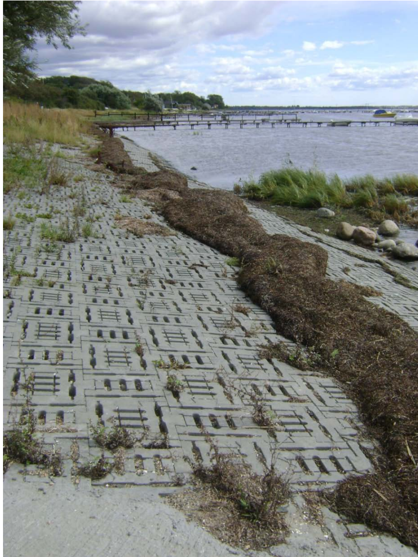
Figure 3.8 Concrete slabs on the shore in Bjärred (2010-09-03)
