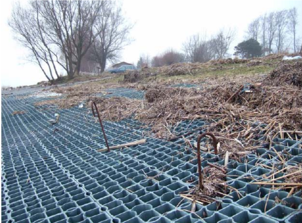
Figure 3.7 Plastic reinforcement nets where macadam has been flushed away (Ramböll, Erosionskydd i Bjärred- utvärdering av skyddsåtgärder, 2007)
