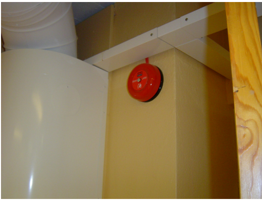
Figure 14. Permanent fire alarm in Sweden (not used in the drills)
