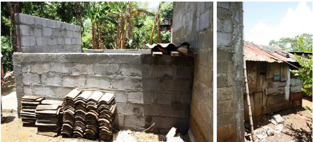
Figure 27. The new storage room is built with blocks of concrete. It is a big difference between the new and the old storage room, which can be seen clearly on the right picture.
