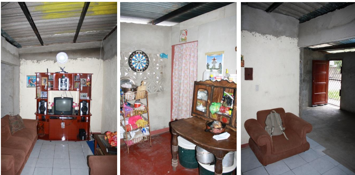
Figure 23. Pictures taken from various angles of the apartment. Common in PRODEL projects is that the clients prefer to add new constructions instead of improving present ones, which is clearly presented in the simplicity of the houses. Notice for example the absence of an under-roof that has a heat isolating effect and prevents the indoor climate to reach extremely high temperatures due to the strong Managuan sun.
