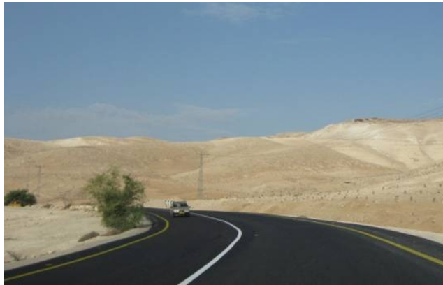
Figure 2.1: Newly paved Main Road. Photo: Lina Eklund 2009
