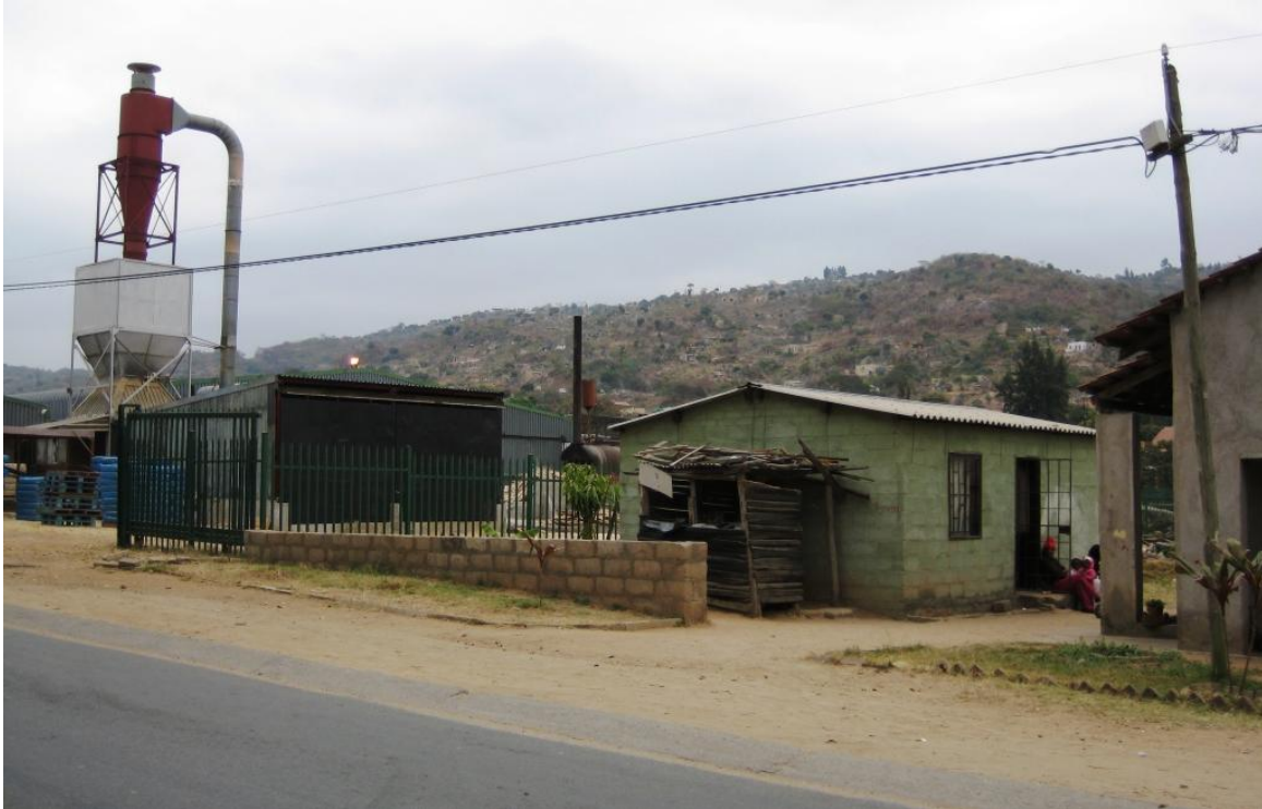
Figure D.1 - Settlements in the presence of an industrial site, Kabokweni.
