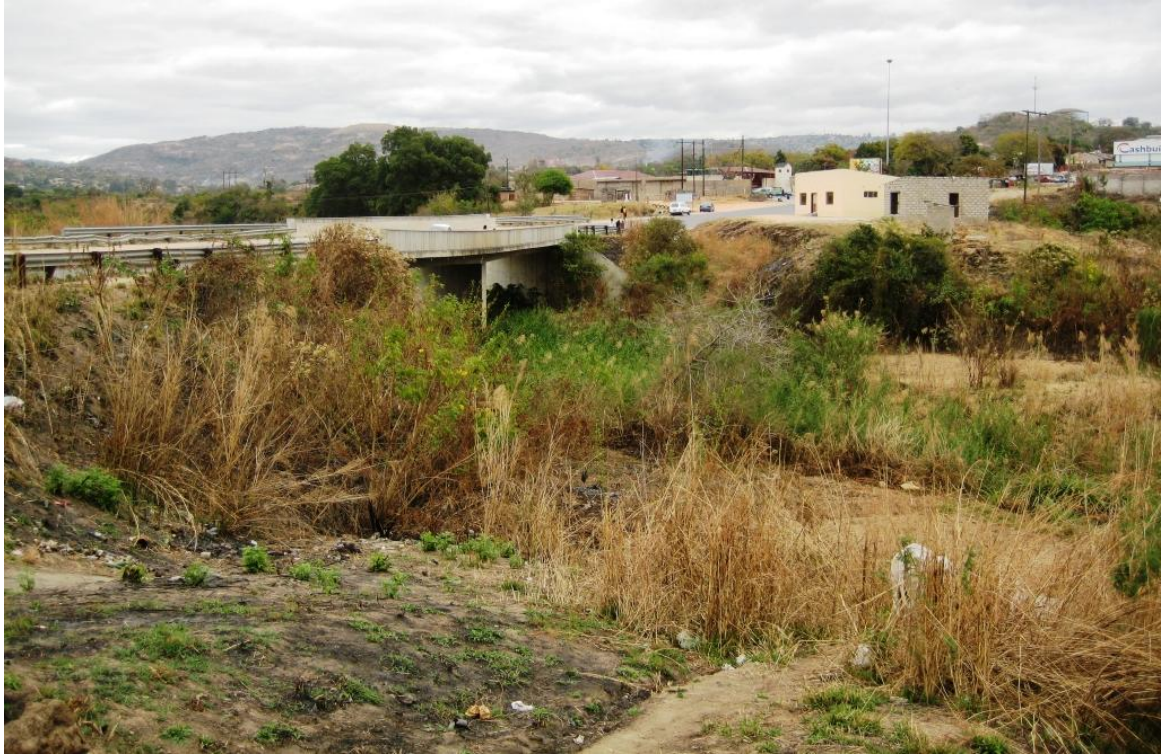
Figure D.3 - Constructions close to the river side, Kabokweni.
