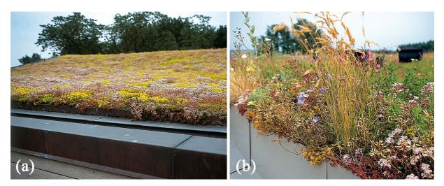
Figure 3. Extensive (a) and intensive (b) green roofs. Source: Veg Tech.
