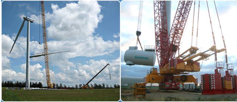
Figure 11. Lifting of blade and nacelle 149
