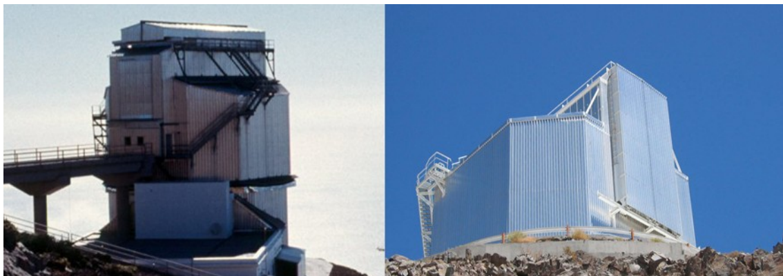
Figure 100. Telescopio Nazionale Galileo, right and NTT , left (showing asymmetric enclosure and space minimization).
