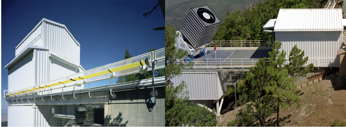
Figure 102. The SDSS telescope and its retractable enclosure. Left photo shows the telescope on day time and right during the observation (photo Princeton University).
