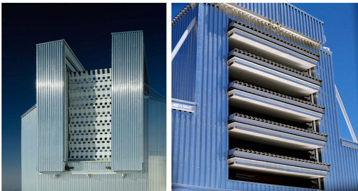
Figure 94. one of a full wind screen, another of a wind-transparent wind screen (photo courtesy ESO NTT).
