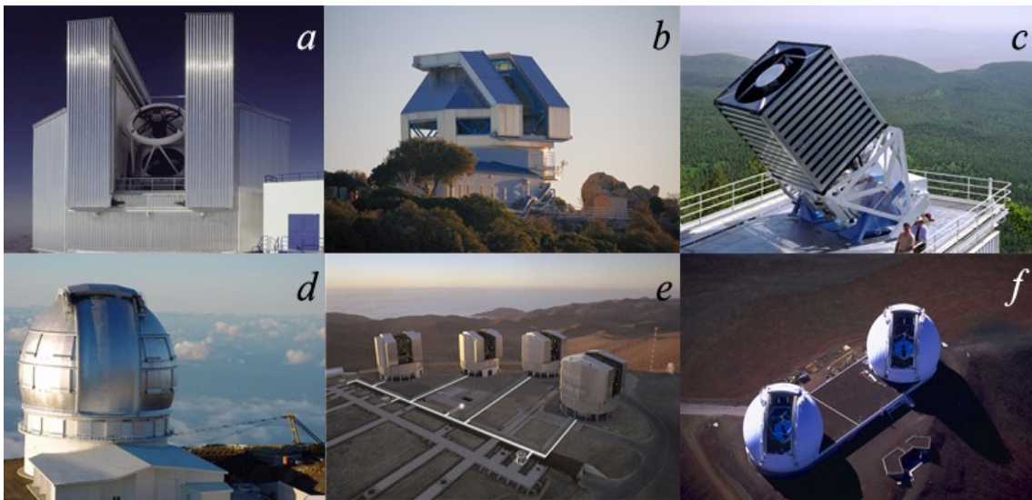
Figure 1. Upper panel: Some modern 3 m class ground based optical telescopes. a) NTT 3.6 m telescope at La Silla, b) WIYN 3.5 m telescope at Kitt Peak, c) Sloan 2.5 m telescope at Apache Point. Lower panel: Some very large optical telescopes, d) Gran Telescopio Canarias (GTC) with a 10.4 m segmented primary mirror at La Palma, e) VLT telescopes at Cerro Paranal, each with a monolithic 8.2 m primary mirror, f) Keck telescopes at Mauna Kea, each with a 9.6 m segmented mirror. (Photos from official websites).
