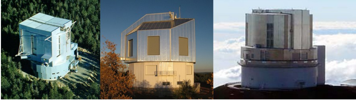
Figure 104. Some telescopes with asymmetric enclosures. LBT at left, DCT at middle, and Subaru telescope at right.
