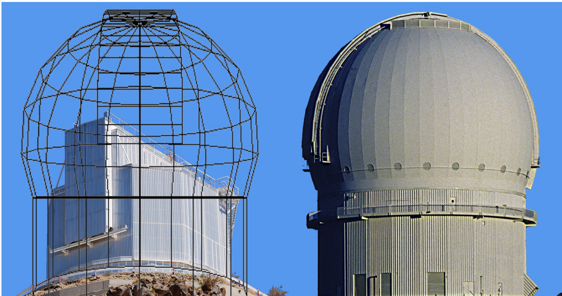
Figure 95. The CFHT telescope enclosure (right) comparing to the ESO NTT telescope enclosure (left). Both telescopes have a 3.6 meter primary mirror but there is a special concern in NTT design for minimizing enclosure inside air volume and at the same time providing enough space for service and maintenance.
