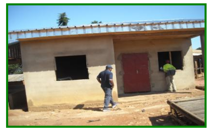
Village Bank at Nkongle, Lebiale Division (under construction)
