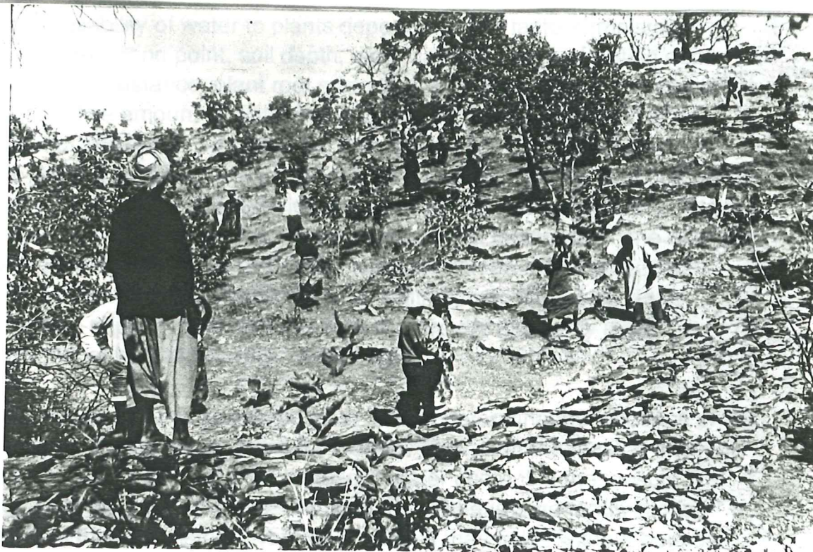
Fig 12. The building of a barrier. (Photo M. Hallberg)
