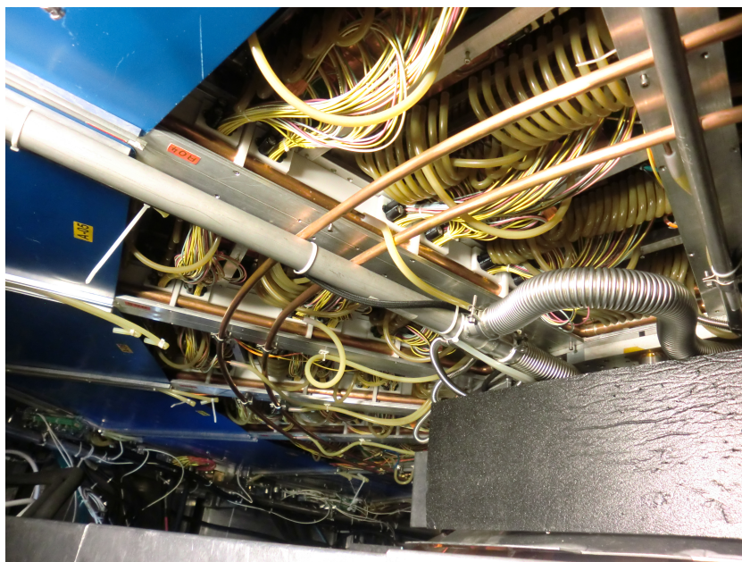
Figure 5.1: Photos taken at P2 on the A-side of the ALICE-TPC during the FEC replacements: The IROC sectors on the A-side of the TPC with the cooling tubes, and low voltage supply for the FEC's.
