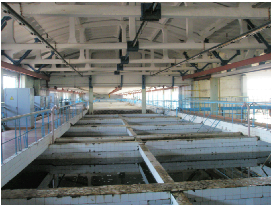
Figure 0-2 Photograph: Sedimentation tanks
