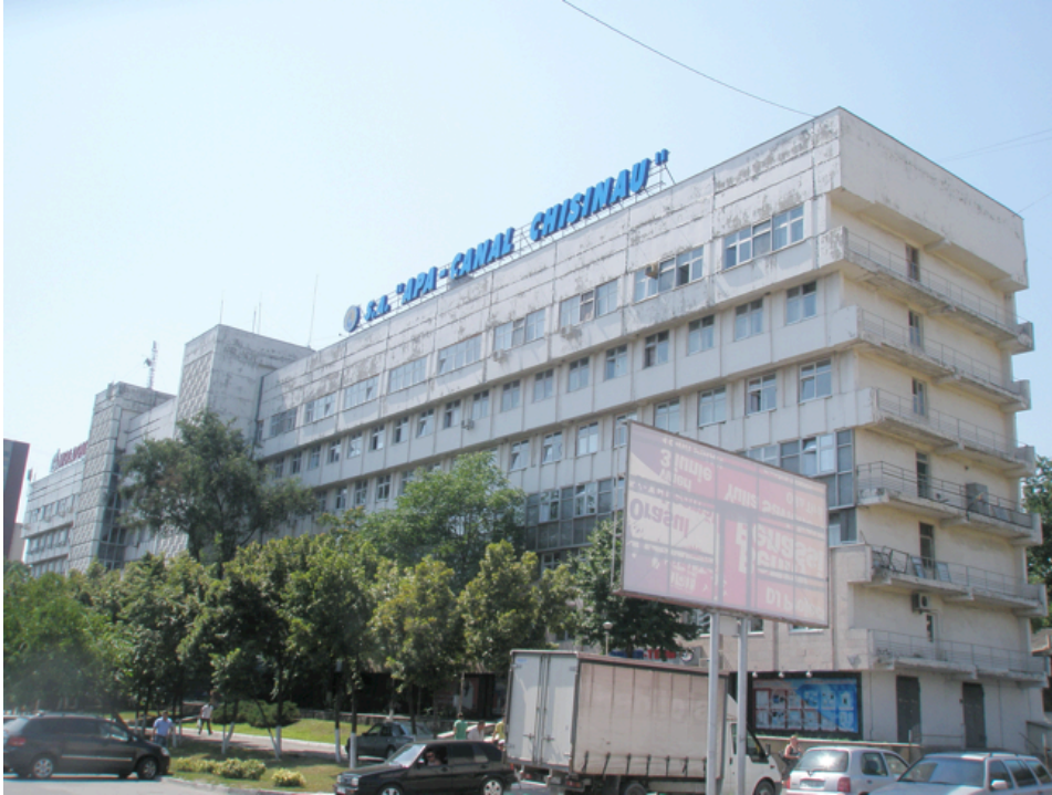
Figure 0-1 Photograph: S.A. Apa- Canal Chisinau Administration building
