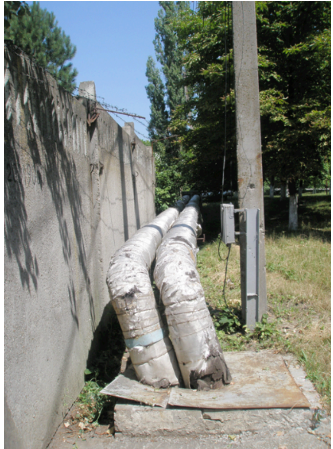
Figure 0-4 Photograph: Water Pipes from the treatment plant to the City
