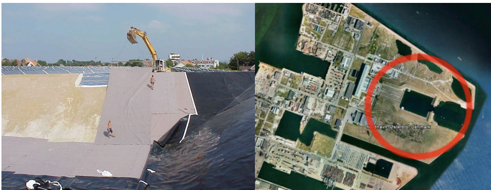
Figure 3-6 'Marstal PTES construction & Proposed North Harbour dry-dock PTES site'
